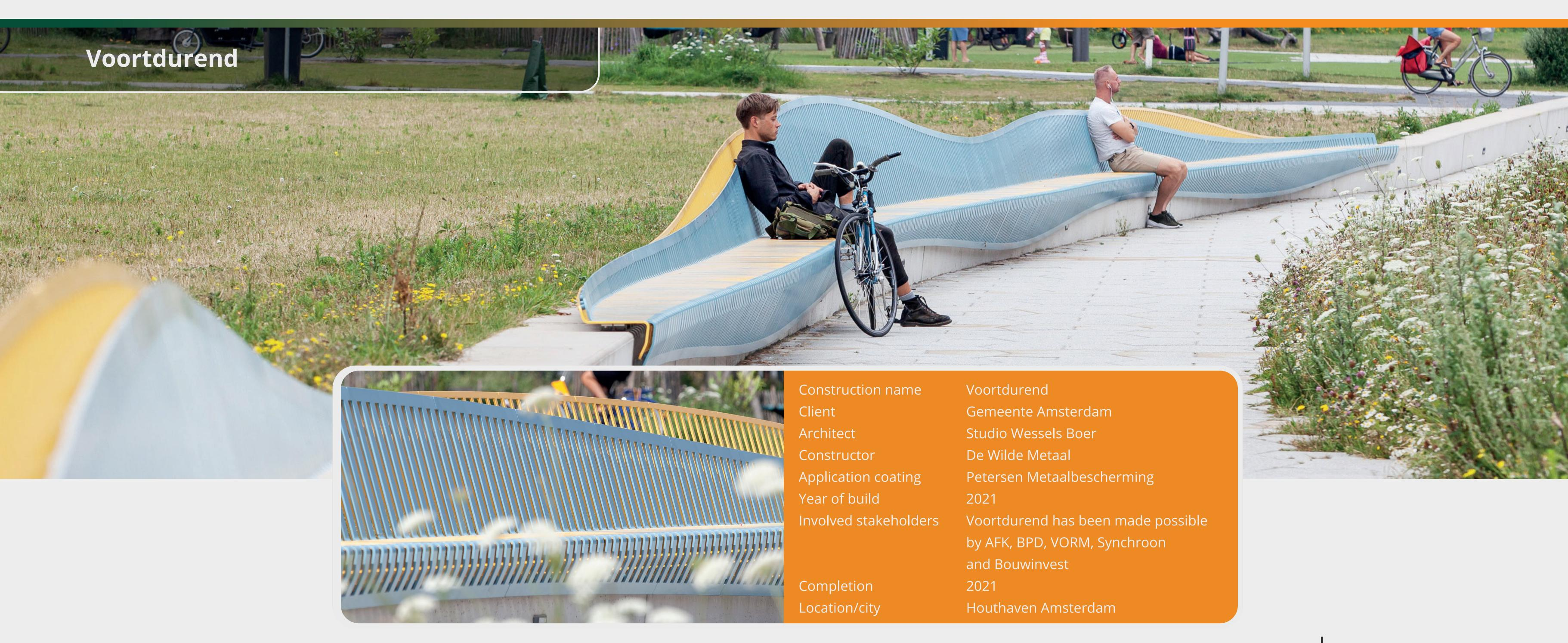
In a park in Amsterdam, that connects two districts, a dike has been excavated. This was an actual old dike which has seen many storms on the sea. The dike has disappeared but what remained was a level difference of the ground. A concrete retaining wall helps leveling the ground. On this retaining wall a 170 meters long seat has been made in the shape of a wave, as a memory of the sea that once was there.
